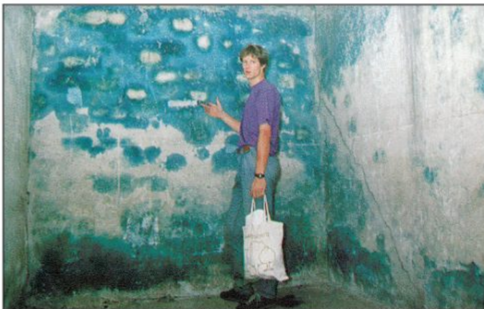
Fig. 69: Picture of a room located in the northwest of the disinfestation wing of building 5a (see Figure 19). The exterior walls are located in the background and to the right, showing intensive blue discolorations caused by iron Blue. Taking locations of samples 9 and 11 are visible. On the left in the picture is the interior wall, erected during the conversion to a hot air disinfestation chamber. Sample 10, with a slightly positive cyanide content, was taken from this wall.
